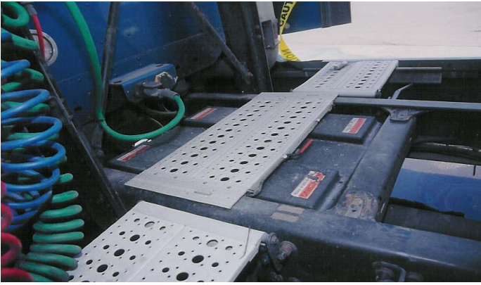
Photo 18 – Battery Access Covers, Freightliner Century Class
