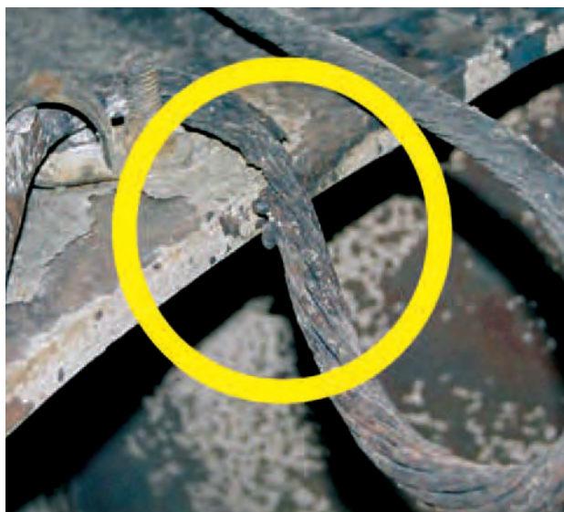
Photo 30: B+ cable contacting structural gusset, creating B+ to ground.
