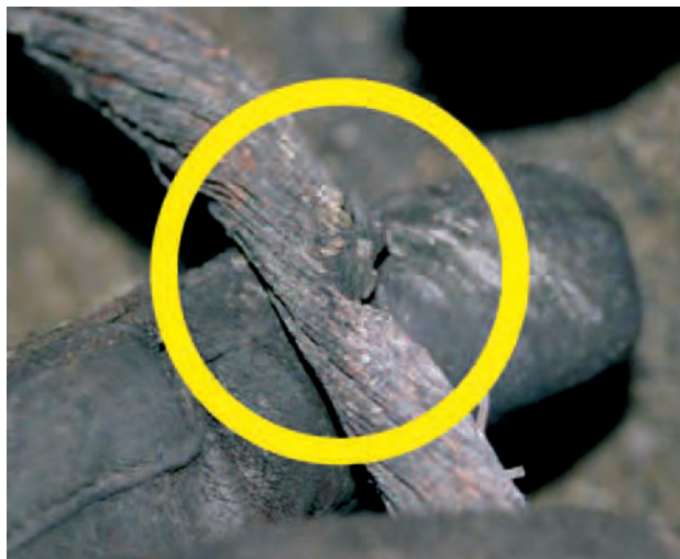
Photo 31: B+ cable with "vee" cut from arcing (same cable as in Photo 30).
