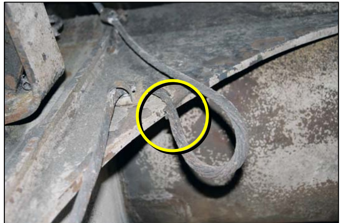
Photo 21: B+ Cable Contacting Structural Gusset Creating B+ to Ground
