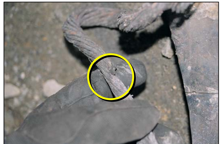
Photo 22: B+ Cable with "Vee" Cut from Arcing (same cable as in Photo 21)
