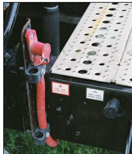
Photo 5A: Remote Jump Posts
