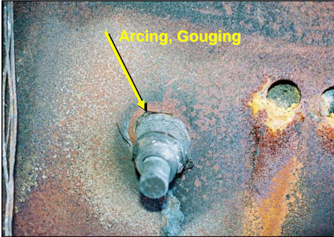
Photo 5B: B+ Jump Post, Battery Box
